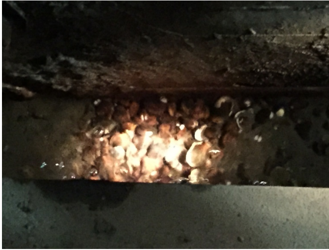
Figure 2. Asian clam shell debris in drainage gallery
