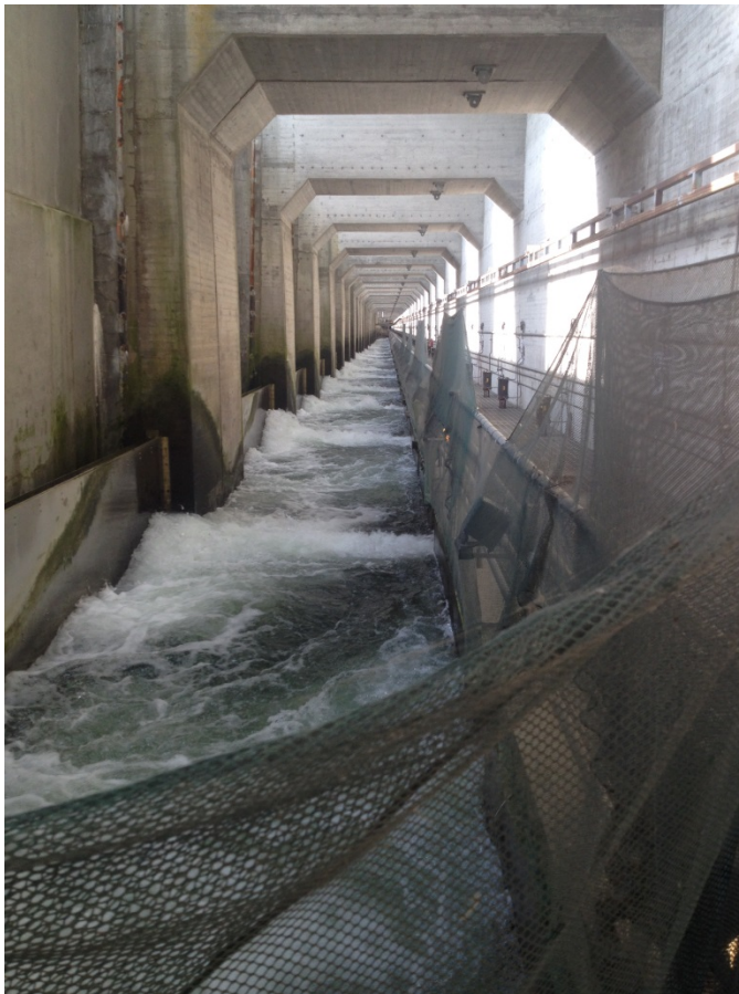
Figure 16. Outfall from orifice at juvenile fish collection channel
