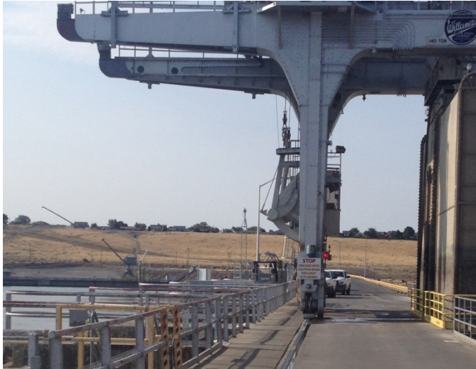
Figure 3. Trash rake
