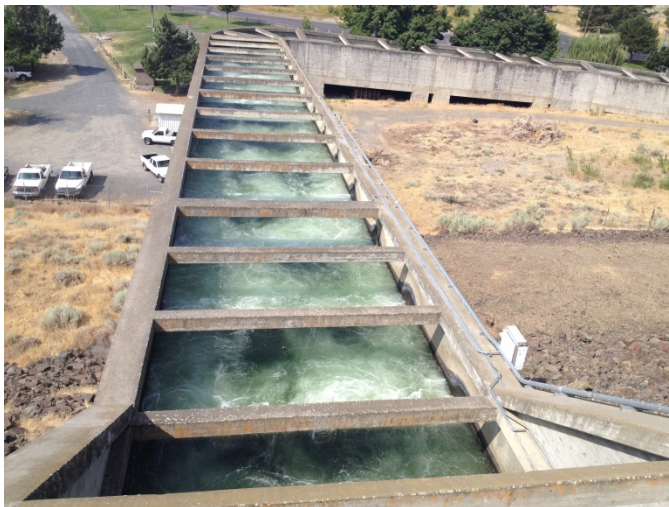
Figure 13. South fish ladder pools
