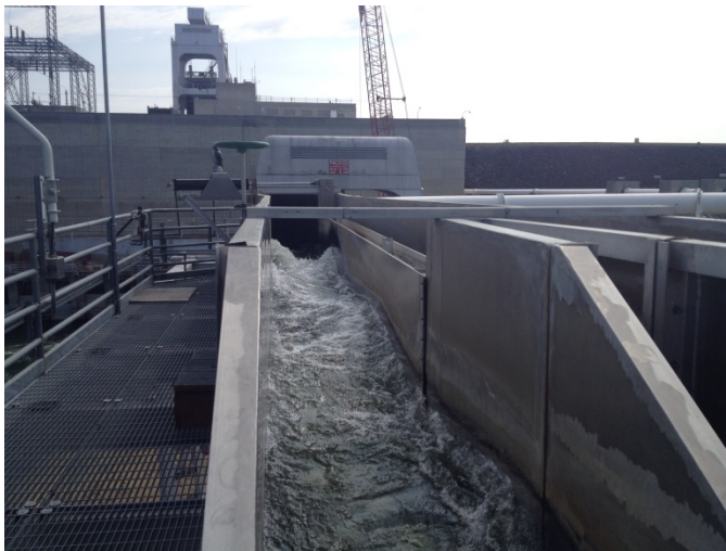
Figure 18. Bypass flume just upstream from JFF
